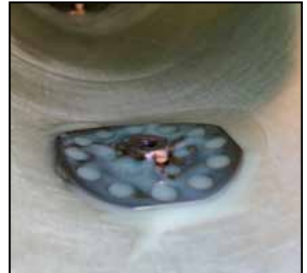
Figure 5: Nut plate installed with epoxy to hold it in place.
