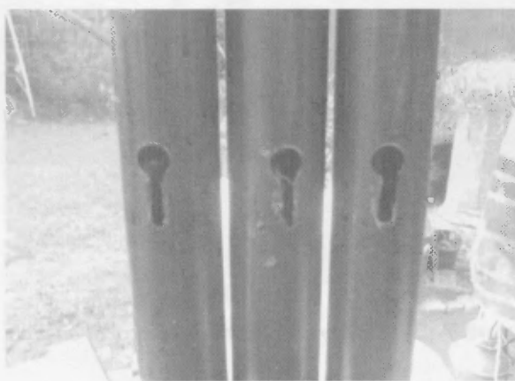
Figure 7-19 The finished set of conduits.
