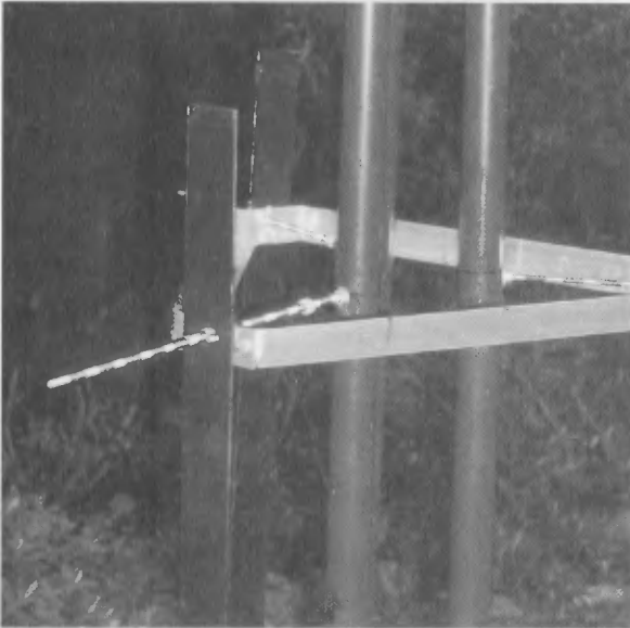
Figure 7-28 Aluminum hexagons bolted to support brackets using threaded rods.
