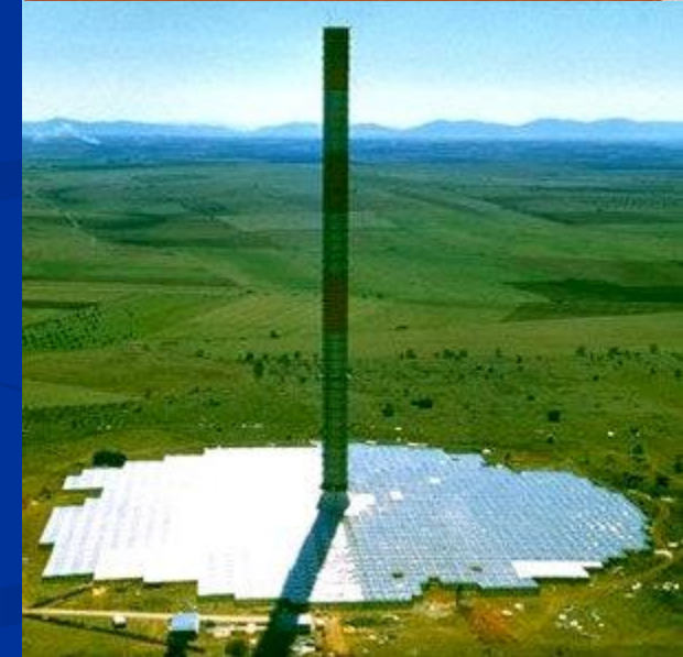
15-MW plant project
