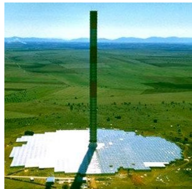
15-MW plant project
